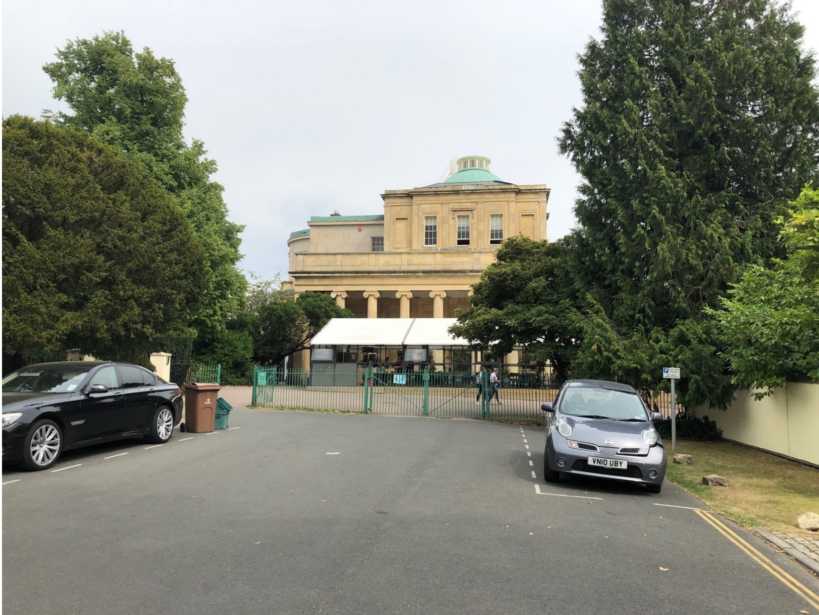
Site photos – View of Orangery when looking east on East Approach Drive
